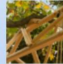
As long as it is in good intent, 2022 installation of different types of wood various sizes
